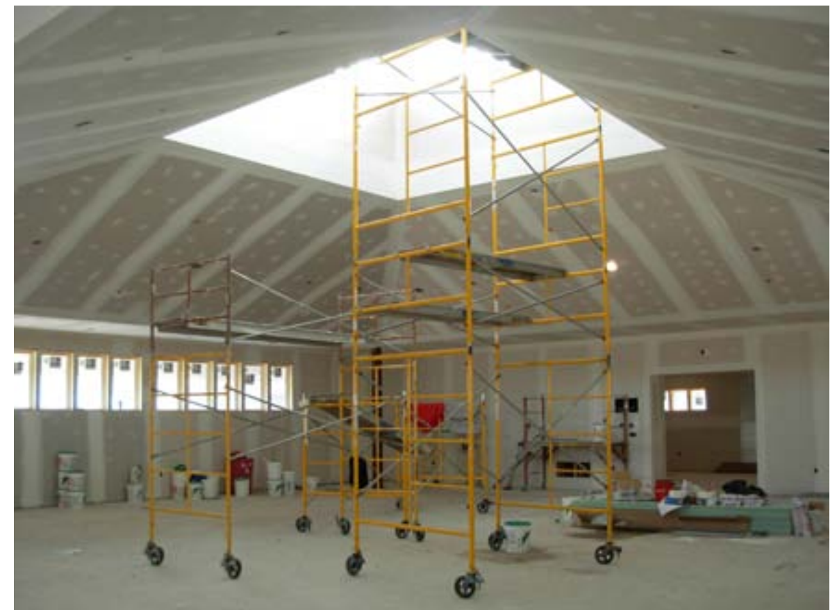
Zendo construction during Phase Two.
